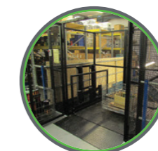
Open cage at mezzanine level
