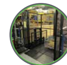
Open cage at mezzanine level
